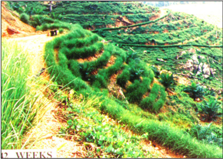
Photo 32a. In Malaysia, vetiver hedgerows stabilize low cost plantation roads at minimal cost and maintenance.
