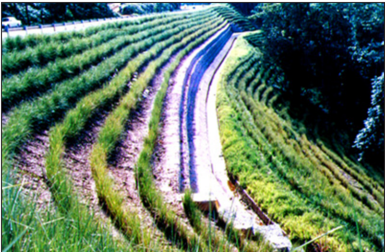
Photo 32b. In Malaysia, vetiver hedgerows stabilize what had been a very unstable highway fill on this high cost expressway.
