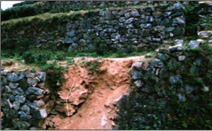
Photo 31. In the Himalayan highlands terraces are frequently washed out by concentrated flows of run-off water.
