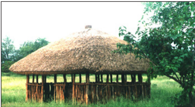
Photo 39. In Zimbabwe, vetiver grass thatch is popular. With good thatching techniques, vetiver thatch will last for many years.
